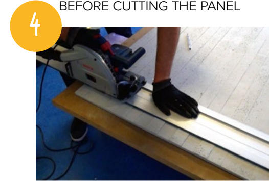
CUTTING WITH THE USE OF A GUIDE RAIL
